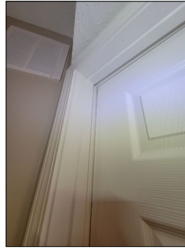
Jambs, primary bedroom
