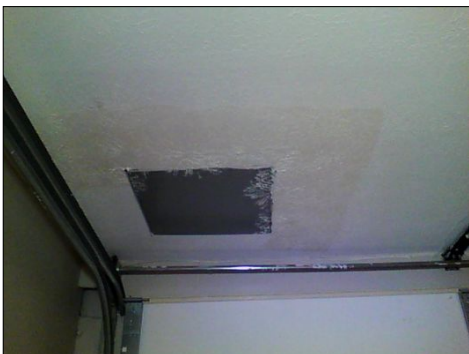
Indicates repair at panel in garage ceiling dry
