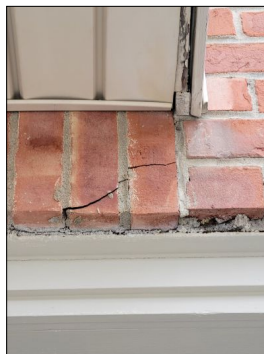
Above garage overhead door
