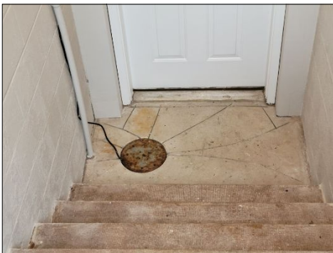
Concrete lines cut for accepting water into sump pump
