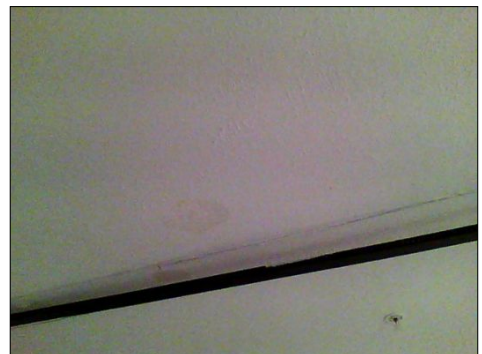
Indicates repair at garage ceiling dry
